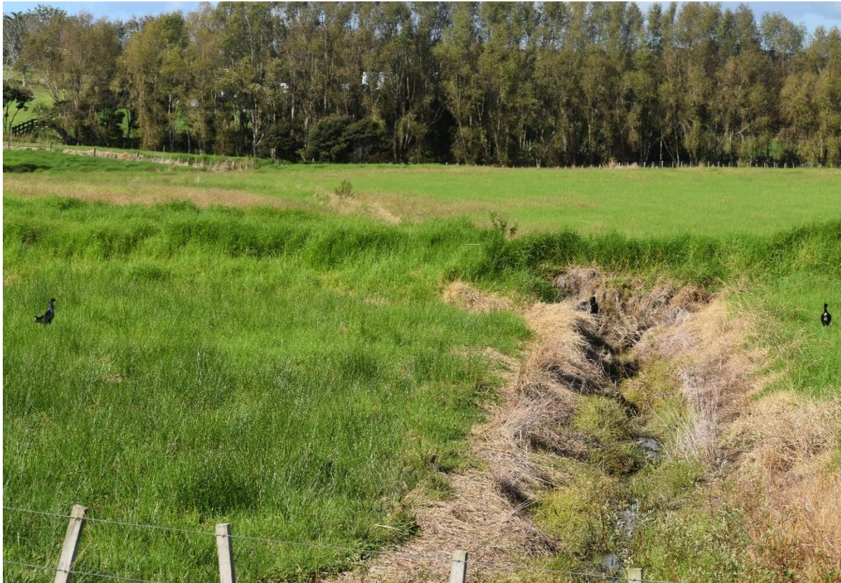
Figure 34: Showing the artificial drainage channel diverting some flows from the intermittent stream towards an existing stormwater pond
